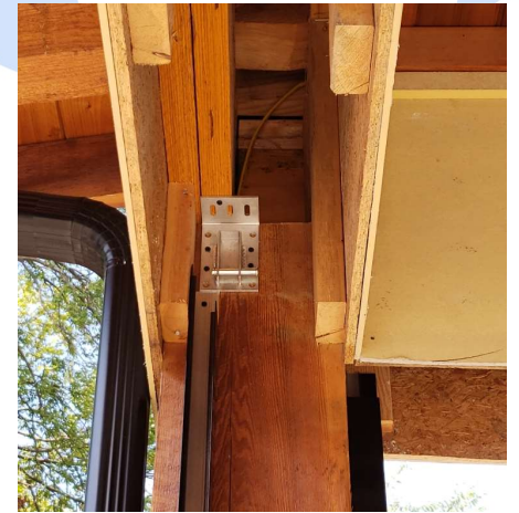
INSTALLATION OF BRACKETS
