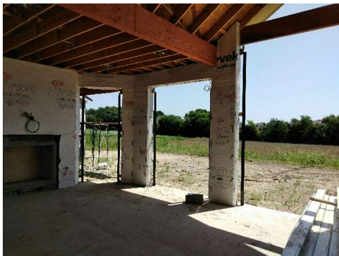
U-CHANNELS INSTALLATION
